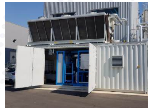
Heat recovery on Incinerator– 180kW ORC - France
