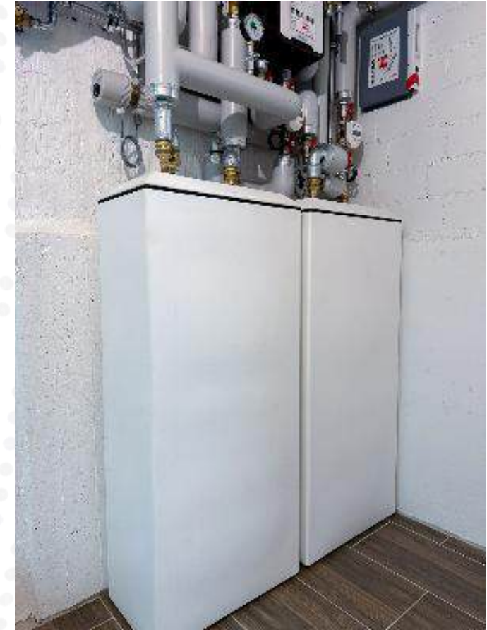
24 kWh of heating and Domestic Hot Water (DHW) storage based on Phase Change Materials.
